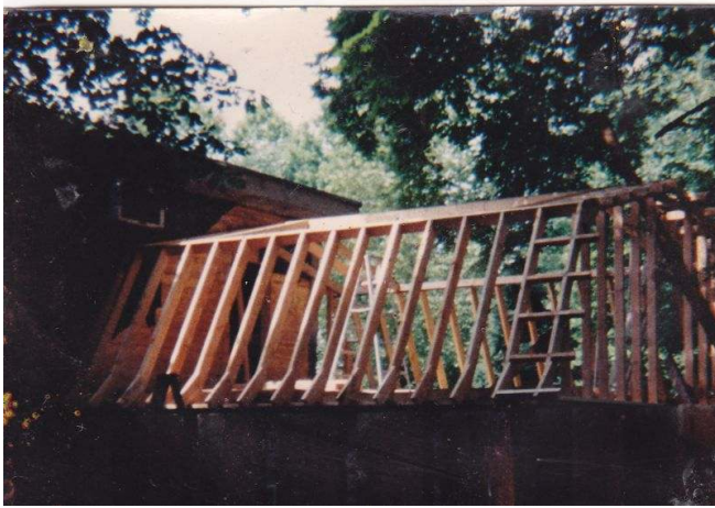
The framing of roof. Then Chris & DMunro putting up the sheathing.
