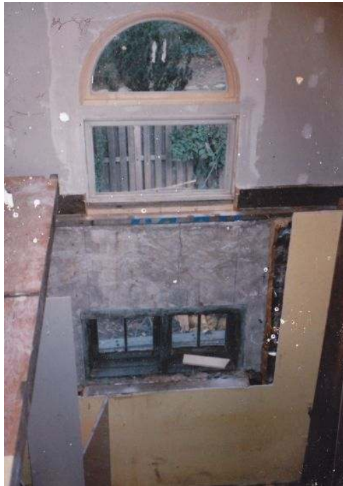
The original window (below) and new one (above)
