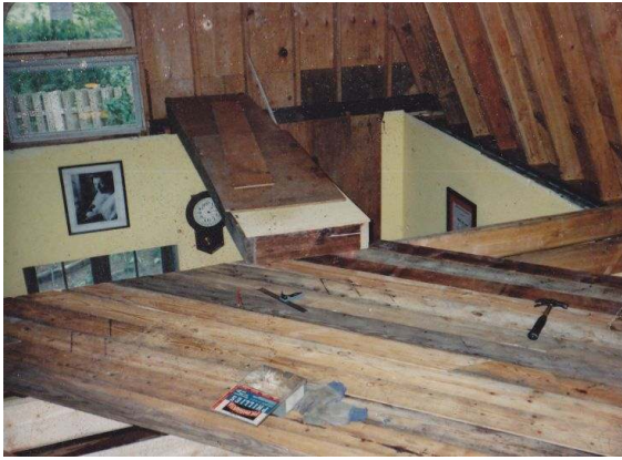
Building the balcony.
