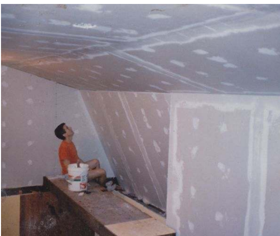
The worst job, plaster-boarding the ceiling.
