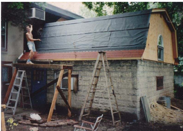
Roof done, beginning shingles.
