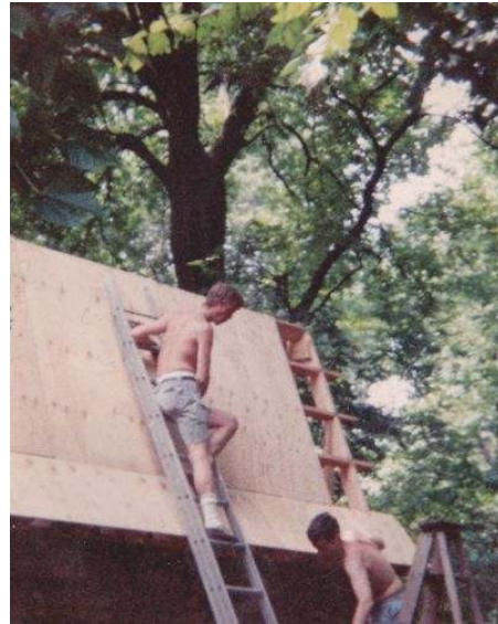
The framing of roof. Then Chris & DMunro putting up the sheathing.
